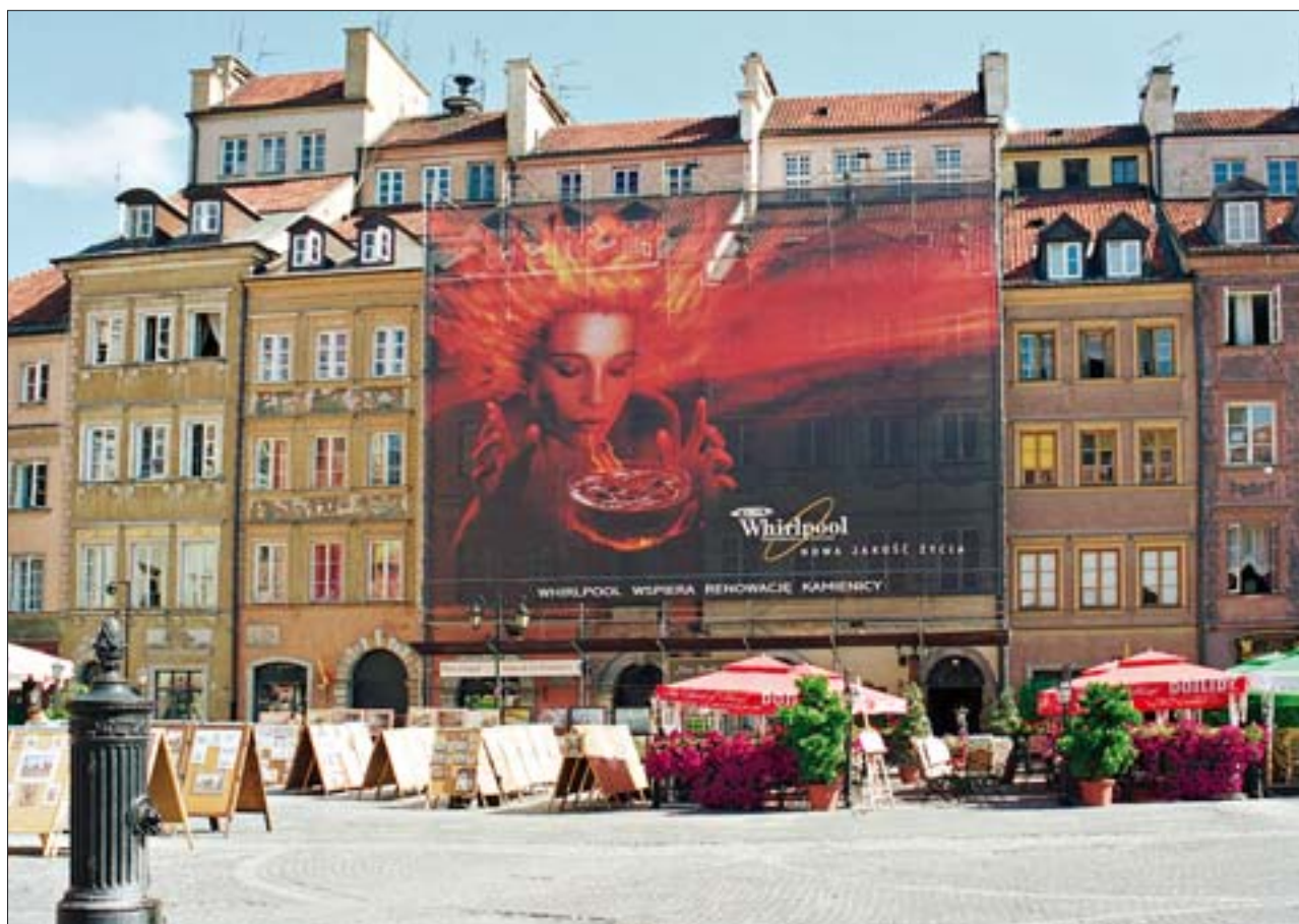
9. Warszawa, remontowane kamienice na Starym Mieście. Fot. archiwum KOBIDZ. 9. Warsaw, renovated buildings in Old Town. Photo from the archives of KOBIDZ.
